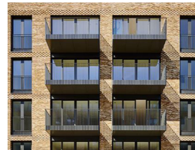
Generous Glazing Proportions and Balcony Detail
